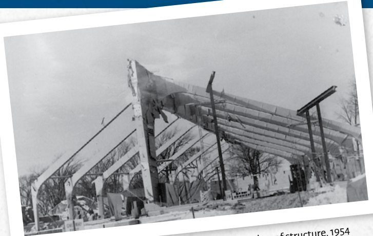
Wood laminated beams installed for new church roof structure, 1954
